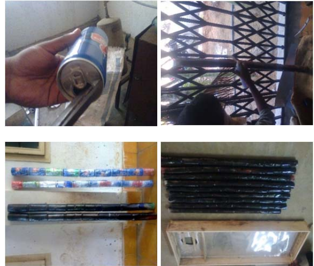
Fig. 5: Coke cans cutting, attaching and painting
